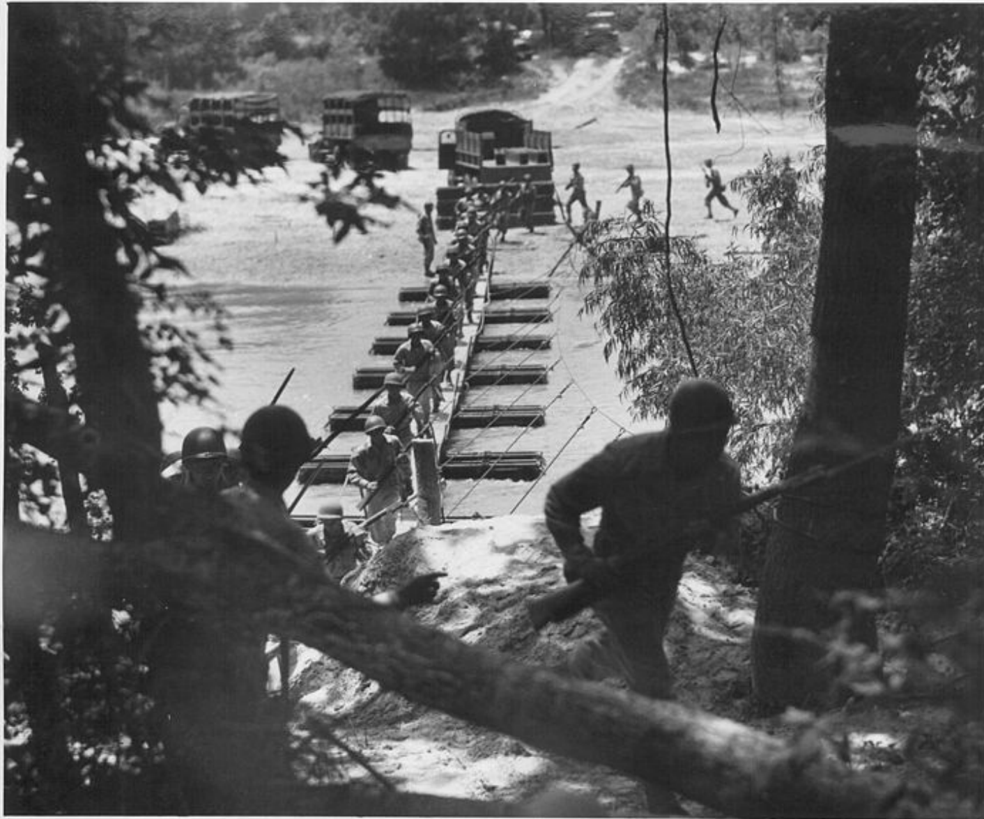
○ Building a pontoon bridge
